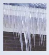
Ice dams are formed when heat from the inside of a home escapes into the attic and warms the roof decking during the winter. This heat, combined with heat from the sun, can melt snow on the roof. Melting snow then runs down toward the eaves as water. When it reaches the cold eaves and gutters, it refreezes.
